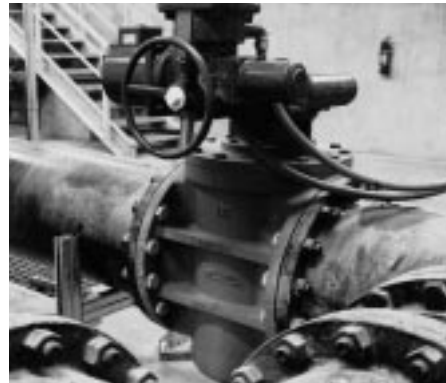
18" motor actuated Cam-Centric® plug valve.
